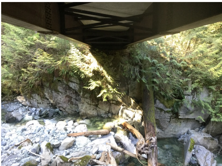
Left Bank Abutment when facing downstream
