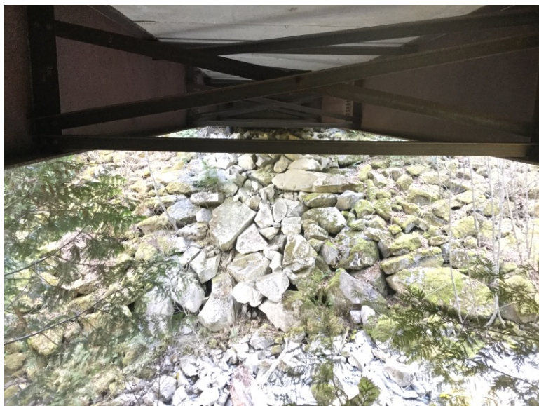
Right Bank Abutment when facing downstream
